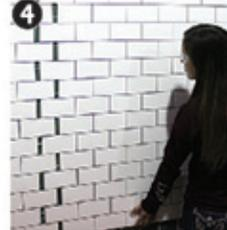
Align the fingerlock joints and press panel to the wall.
