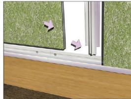
Step 2: Using Marlite adhesive, install the panels and selected vertical reveal.
