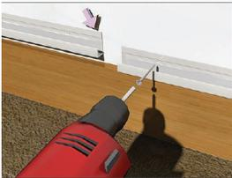
Step 1: Attach LP570 Edge Cap at bottom of installation and as perimeter trim.
