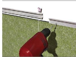
Step 3: Secure the panels and attach desired horizontal reveal.
