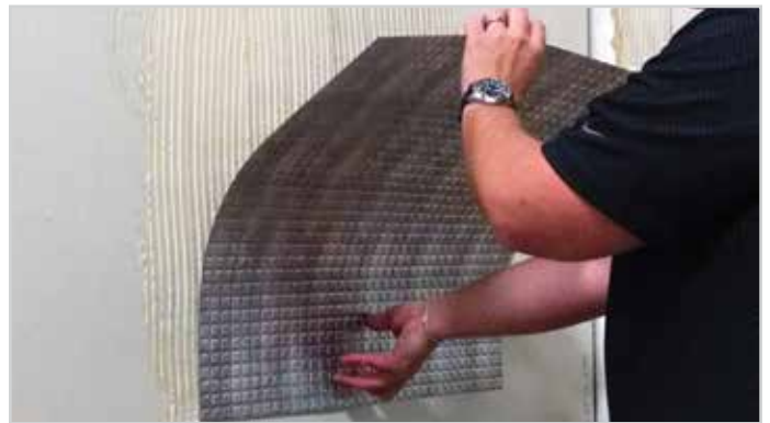
Starting with the bottom of the panel, apply to the wall.
