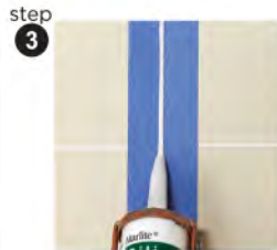
Place a bead of harmonizing sealant in the gap.
