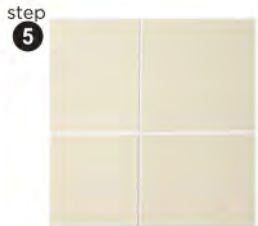
Remove tape to reveal a grooved and matched seam joint.
