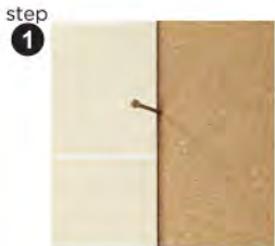
Place a 6 Penny spacing nail between panels.
