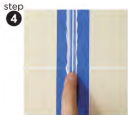
Using your finger, place a slight indentation in the gap.
