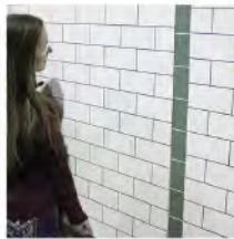
Apply Panels to a prepared subwall.
