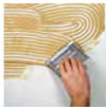
Apply Marlite Brand Adhesive to the back of panels.
